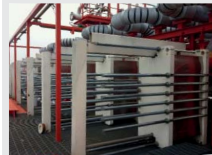
APV Semi-welded plate heat exchangers as main propane pre-heaters and evaporators integrated in Hamworthy Oil & Gas Systems AS regasification module on FSRU Vessel Khannur owned by Golar LNG. Photo courtesy: Hamworthy Gas Systems AS
