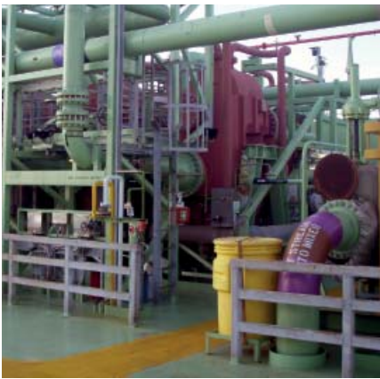
APV Hybrid welded plate heat exchangers operating as wet crude heaters on board BW Offshore FPSO Yuum K'ak Náab in operation for Pemex. Photo courtesy BW Offshore.
