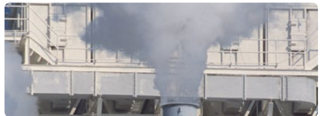
Free cooling, Heat recovery, Water Source Heat Pump, Thermal Storage, Pressure Interceptor, District Heating & Cooling
